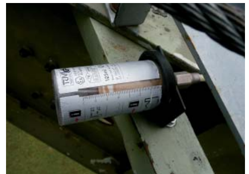
simalube ® lubricates the carrying cable of the Gemmi cable car at each pylon.
