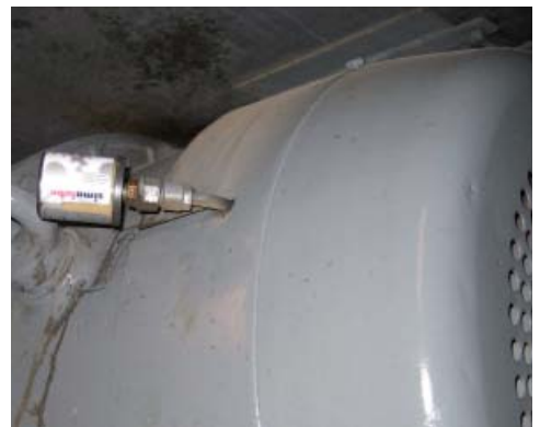
simalube ® attached to a ventilator motor horizontally.
