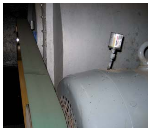
A 60ml dispenser attached to a ventilation motor.
