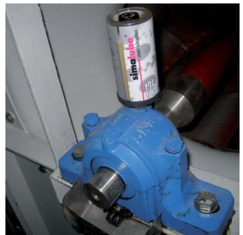
125ml simalube ® dispenser installed on a plummer block.
